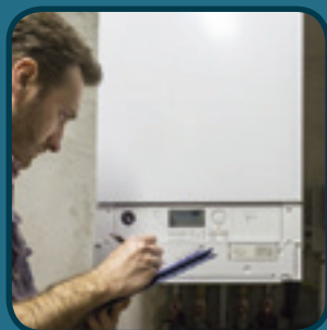
Protects boilers & equipment
